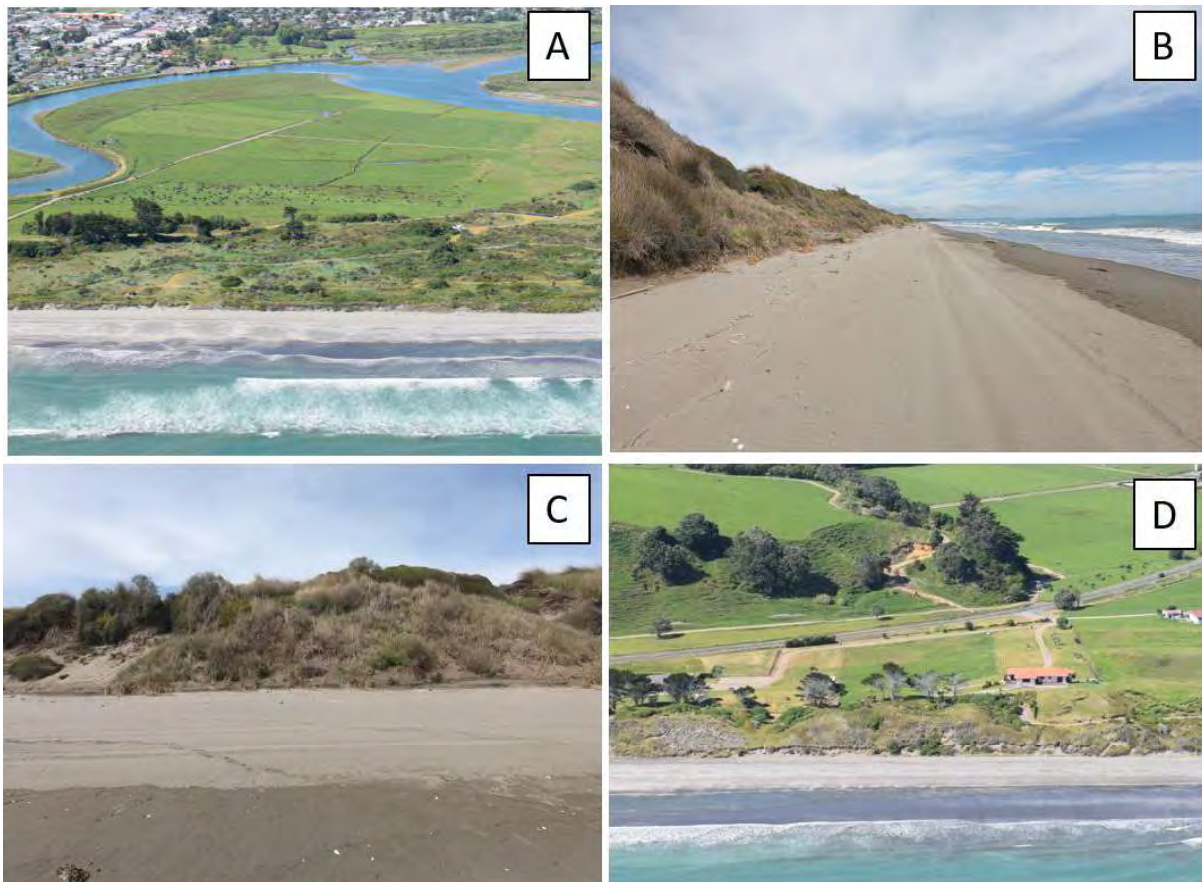
Figure 2.2: Site photos along Hikuwai beach (A) Cell 2A, (B), Vegetated dune within Cell 2A, (C) Vegetated dune within Cell 2B, (D) aerial view of Cell 2B
