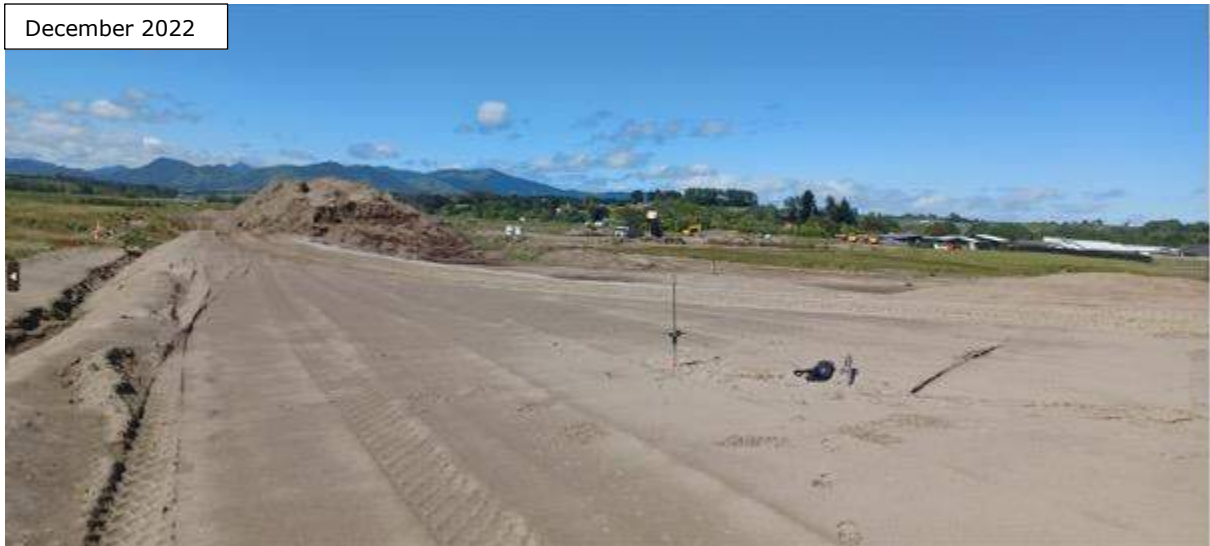
Figure 7: Compaction Inspection Lots 37 – 41
