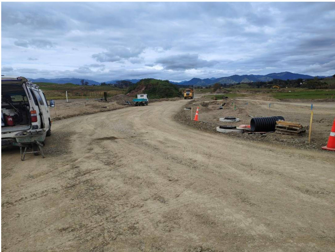
Photo 5: Stage 6C road, looking south east
