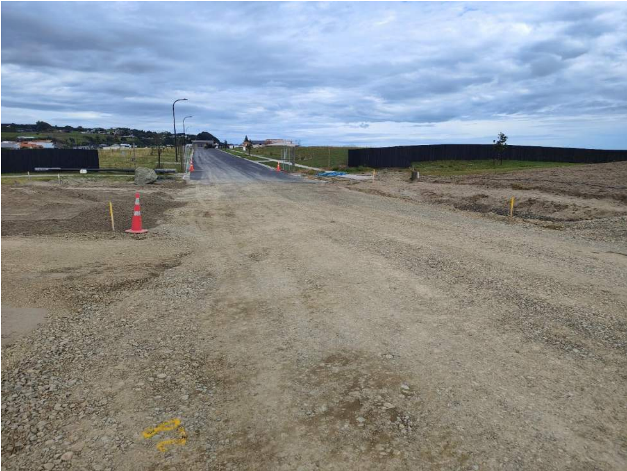
Photo 3: Stage 6B Road, looking west
