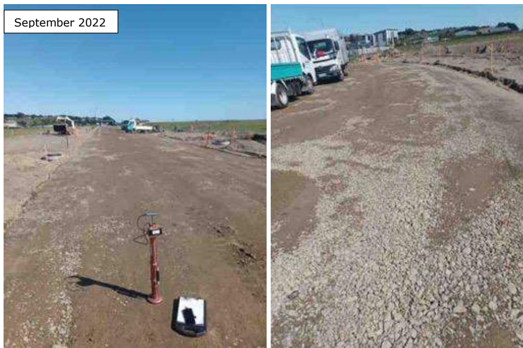
Figure 10: Subbase investigation for Stage 6C
