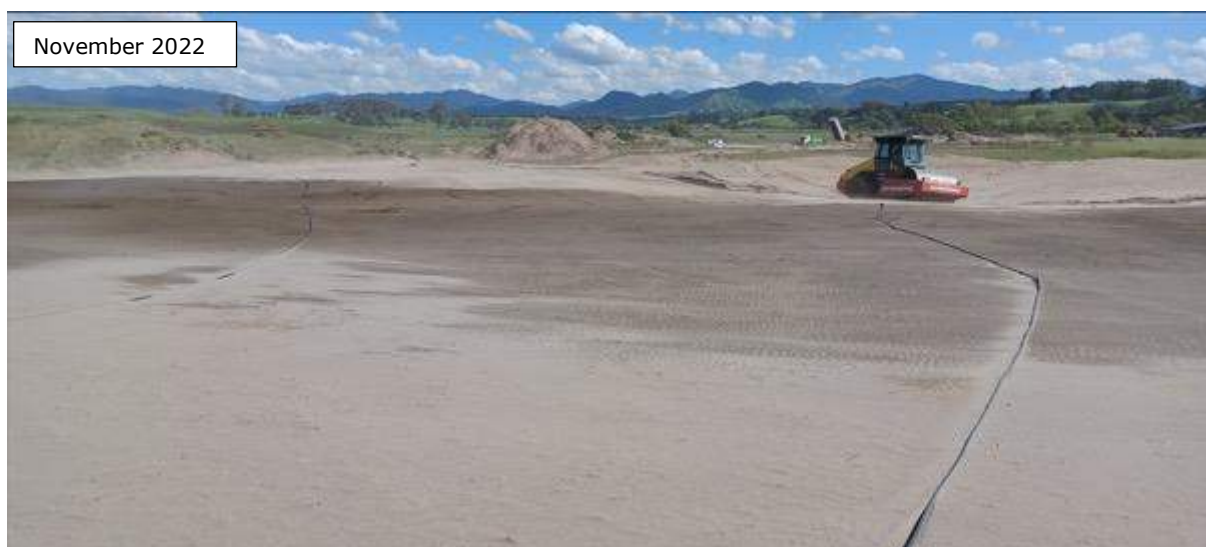
Figure 6: Compaction Inspection Lots 31, 32, 35 & 36
