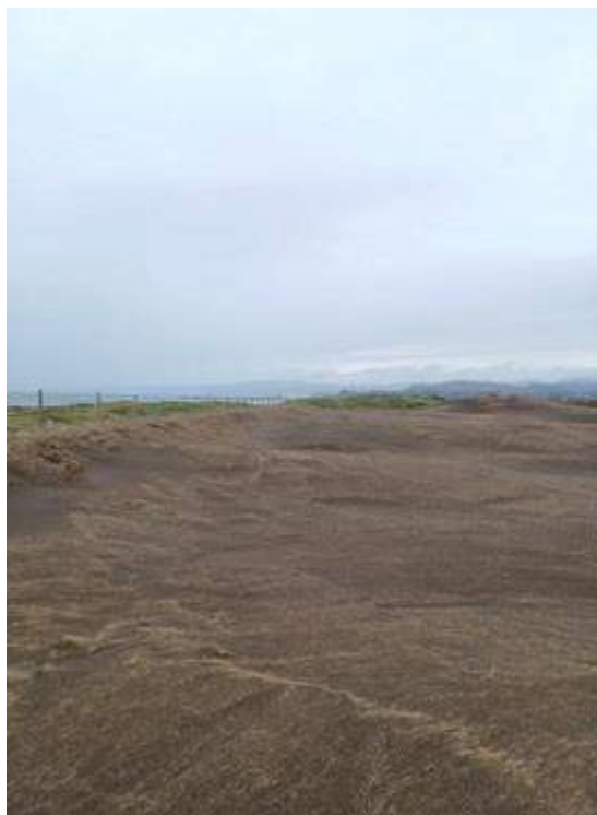
Figure 5: Formation inspection for Stage 6C
