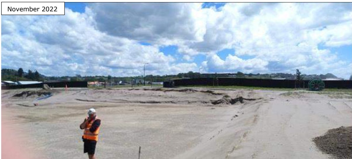
Figure 6: View Lots 25 & 26 being filled with river run.
