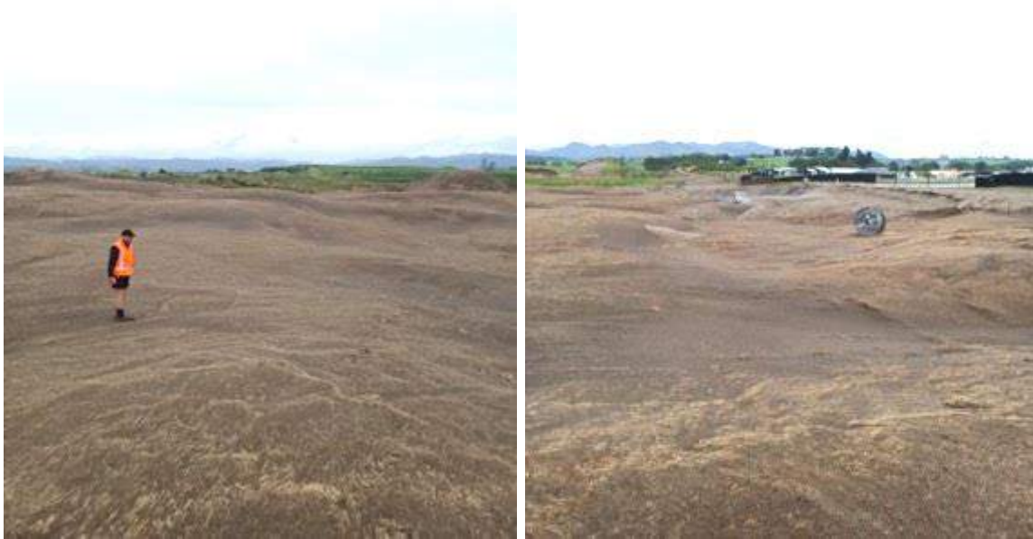
Figure 5: 1 st Formation inspection for stage 6B
