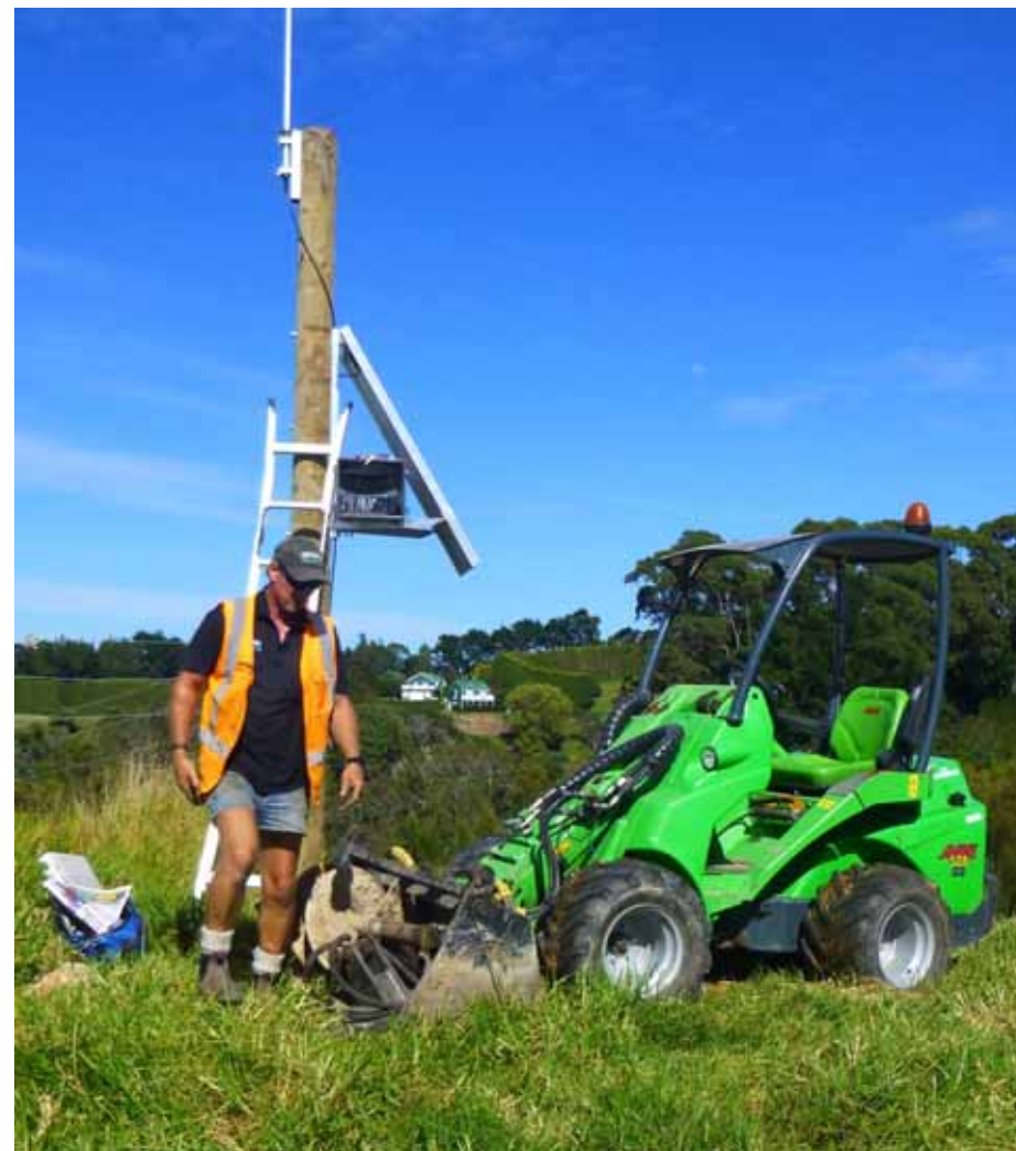
Image: A contractor installs a new Emergency Management telecommunications repeater
