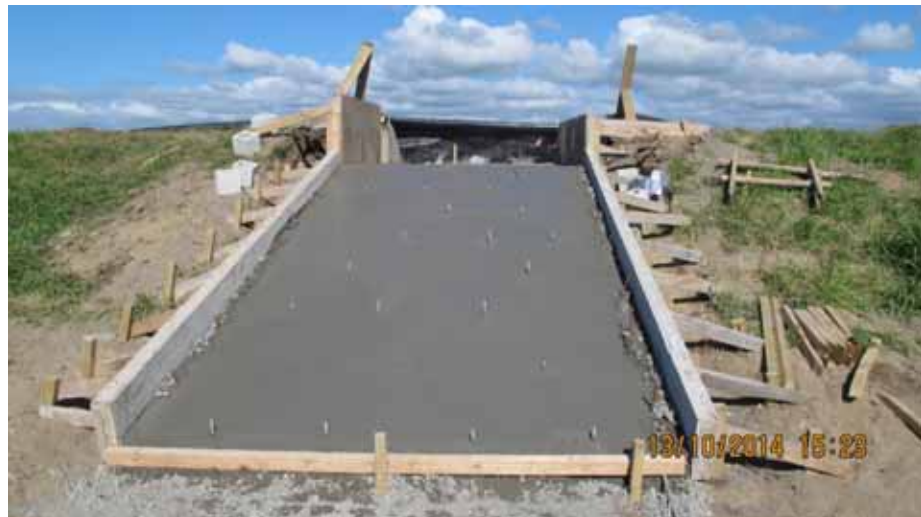
Image: New Weir for Sewer Pond
