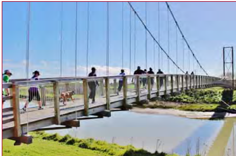
Image: Pakowhai ki Otutaopuku Bridge, Opotiki
