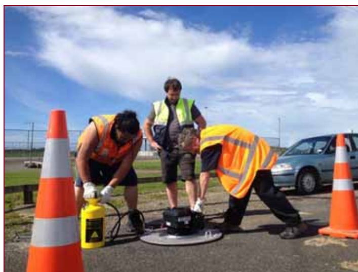
Image: Testing of Ōpōtiki Sewage connections
