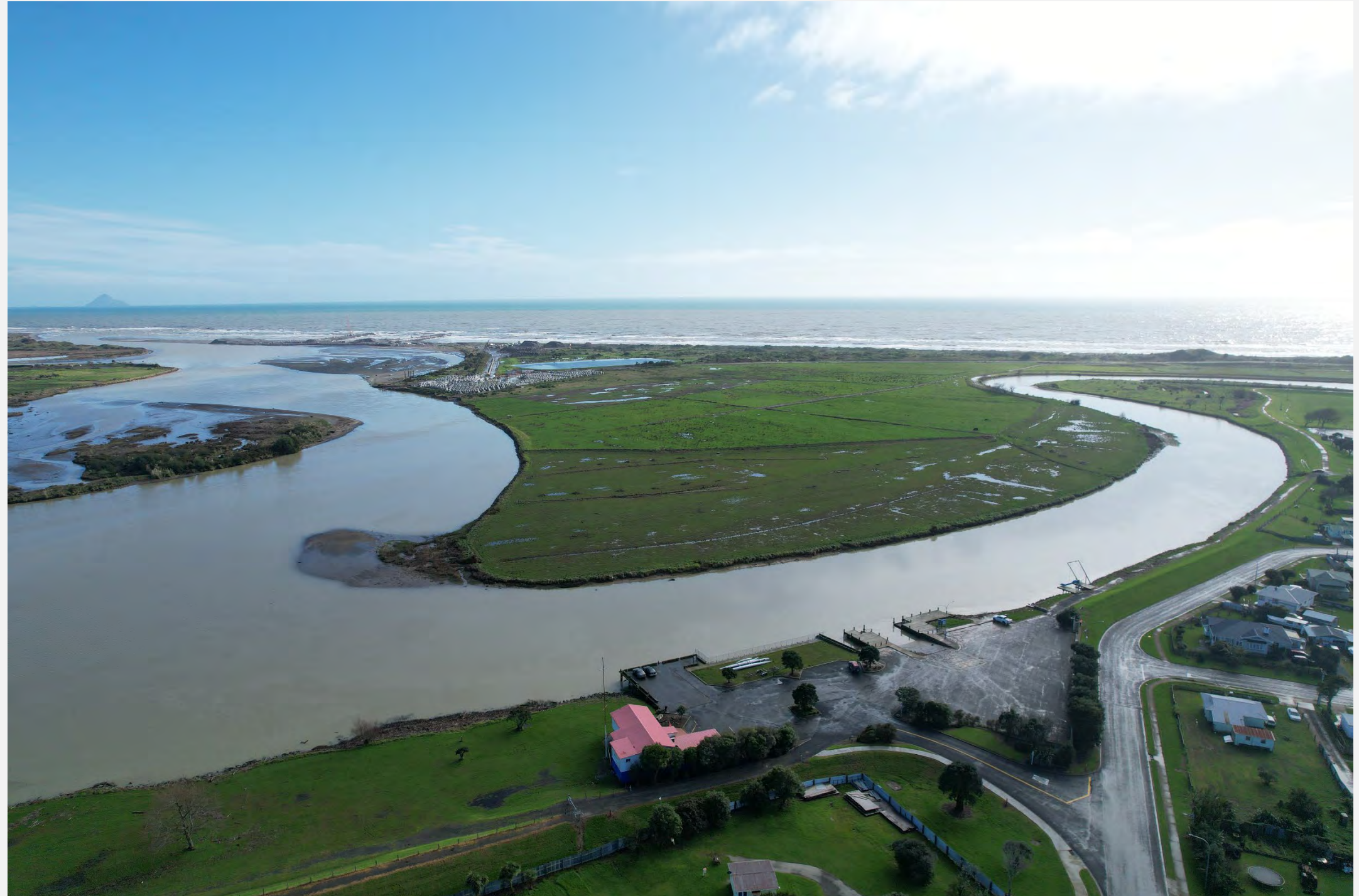
Figure 9: Drone photo of existing wharf and proposed site for new ramp and associated facilities, Snell Road (supplied by ŌDC)
