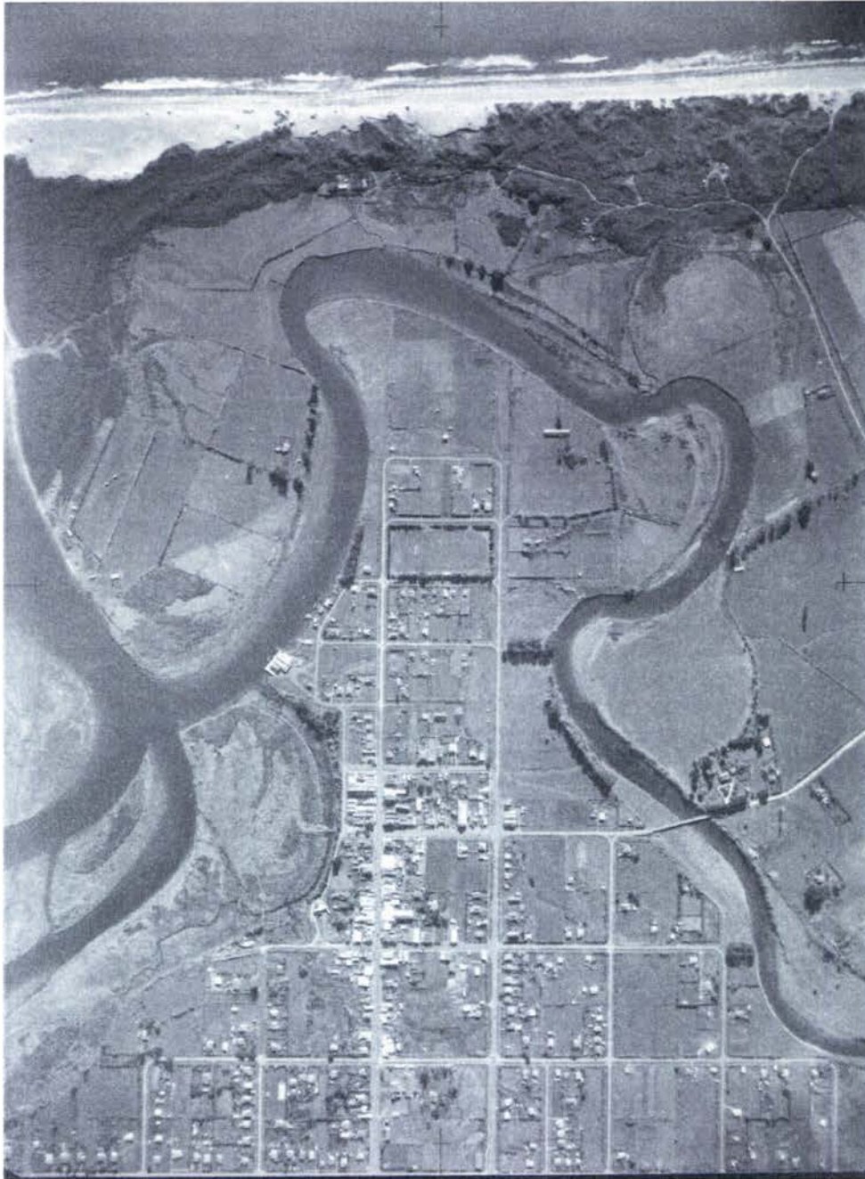
Opotiki is situated on flat land within a loop of the Otara River which flows on the east, north and northwest of the town then merges with the Waioeka River which flows on the west of the town. Until a few decades ago, a side channel of the Waioeka flowed much closer to the town (beside Potts Avenue) around a low-lying island, but as this photo shows, by 1947 this channel had almost filled in. The two tidal rivers together form a natural harbour which opens to the sea about 1 km away. Copy of aerial photo dating from 1947.
