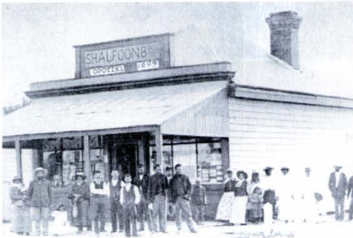
Shalfoon Bros Store on the corner of Kelly Street and Church Street is one of the earliest and most enduring family businesses in Opotiki. Opotiki District Council Photograph archive, Vol 2, 24.
