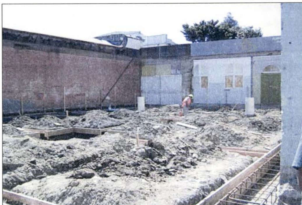
Figure 2. Ground disturbance associated with the Opotiki Museum development. C. 1900 historic artifacts were disturbed during the excavation of foundation trenches.
