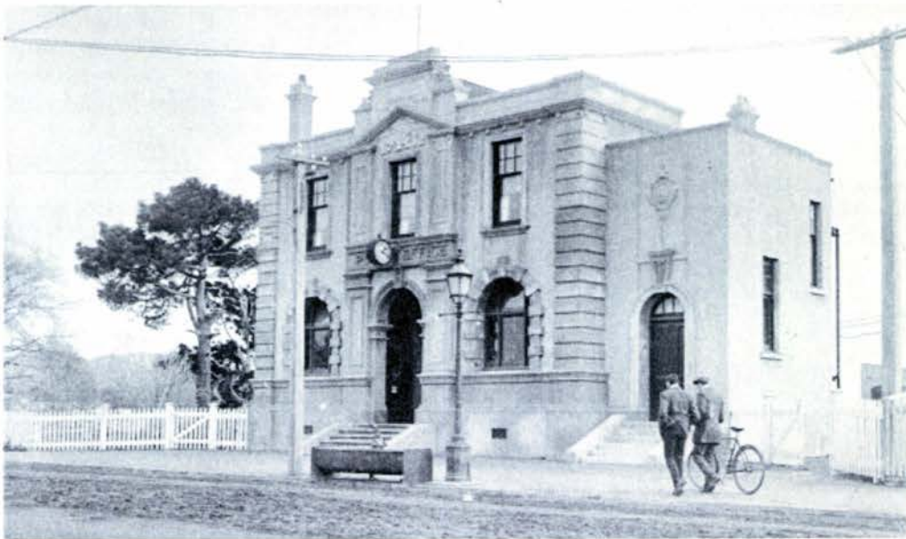
The grandeur of the new Post Office reflects its role in the district. Opotiki District Council Photograph Archive , Vol 2, 218.
