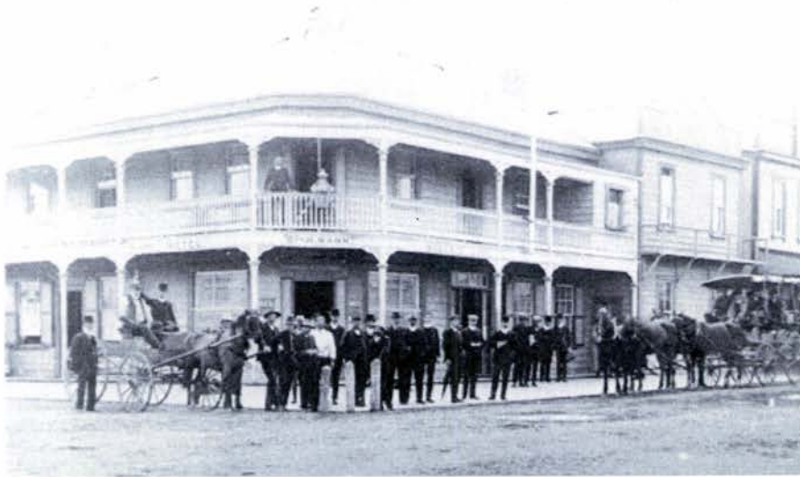
The first Masonic Hotel on the corner of Elliott Street and Church Streets was typical of many Victorian timber hotels around New Zealand. The buildings adjacent also indicate typical early commercial development in timber construction. Fire was a constant threat, and after 1913 the Borough Council made it a requirement to build in permanent materials in the town centre. Opotiki District Council Photograph Archive Vol 1,174.
