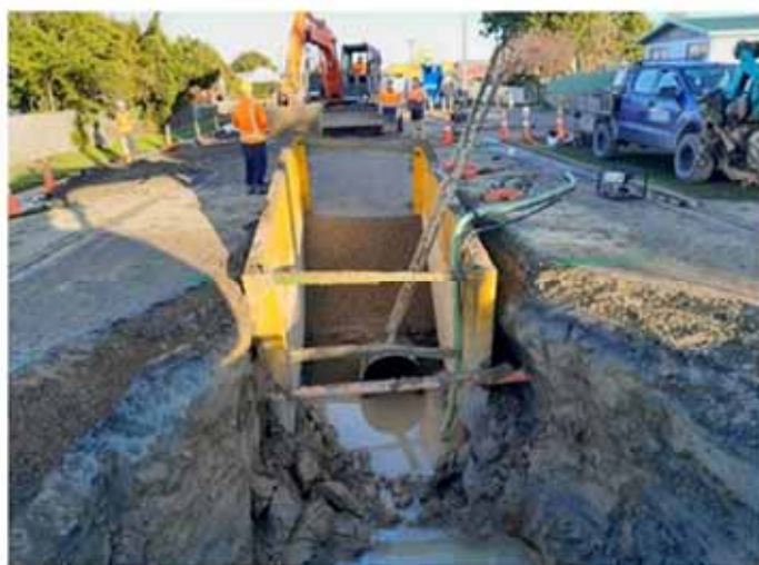
Image: Laying stormwater pipe Richard Street, Ōpōtiki
