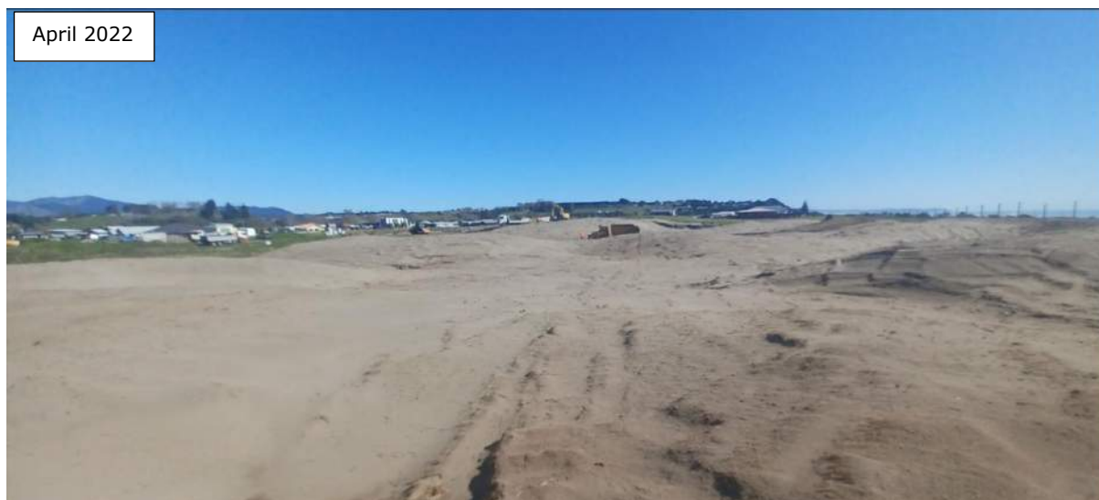
Figure 5: 1 st Formation inspection for stage 5B
