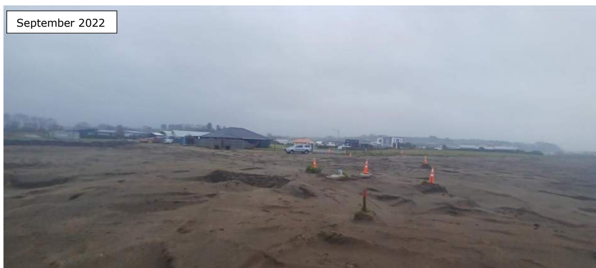
Figure 11: Compaction Inspection for Stage 6A
