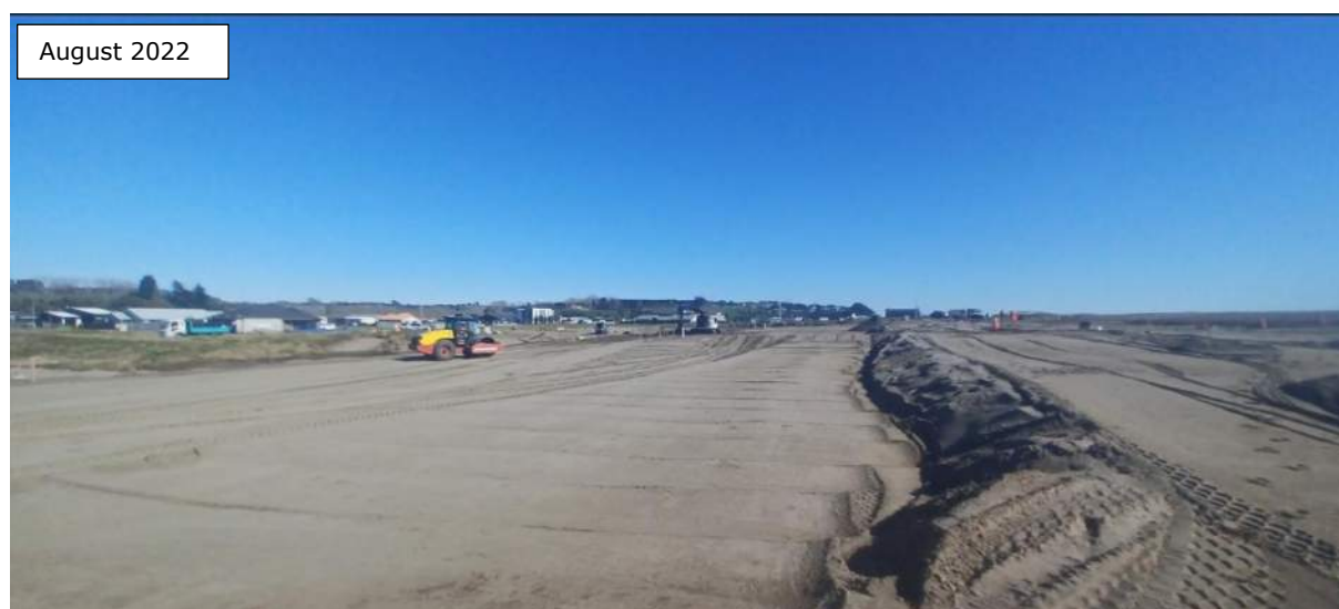
Figure 8: 2 nd Compaction Inspection for Stage 5B
