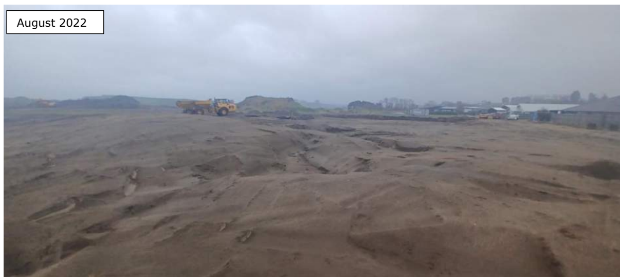
Figure 10: Formation inspection for Stage 6A
