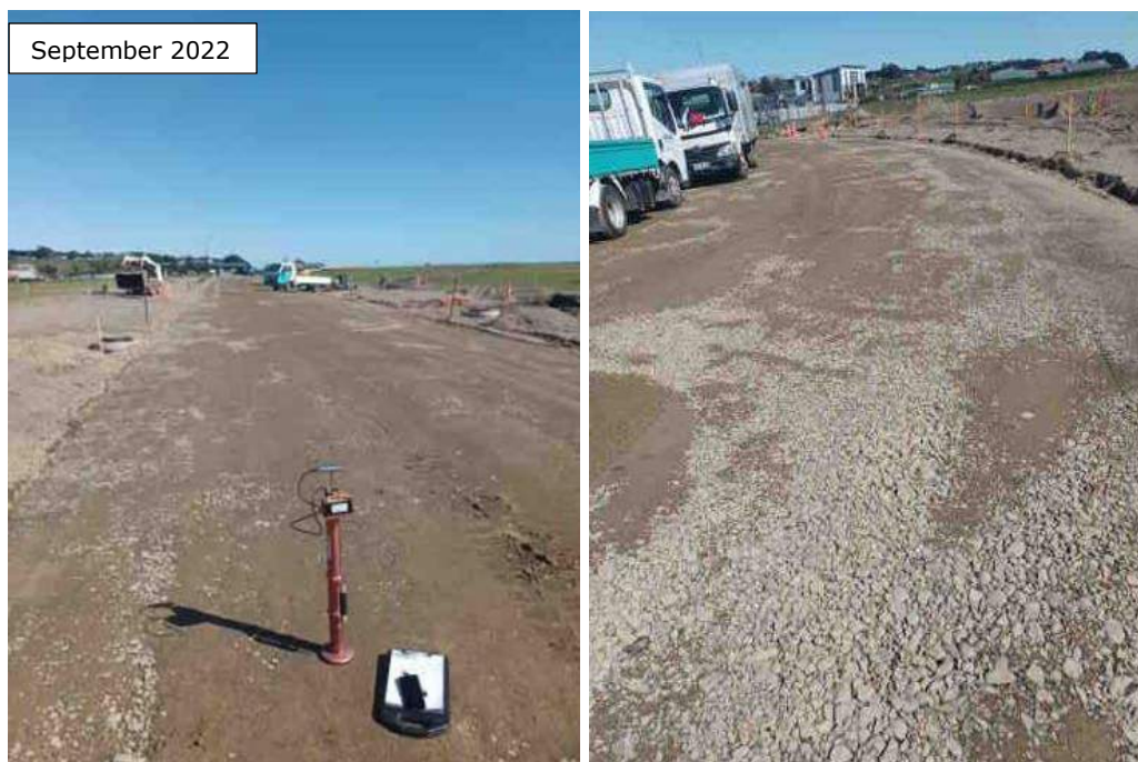
Figure 12: Subbase investigation for Stage 6A
