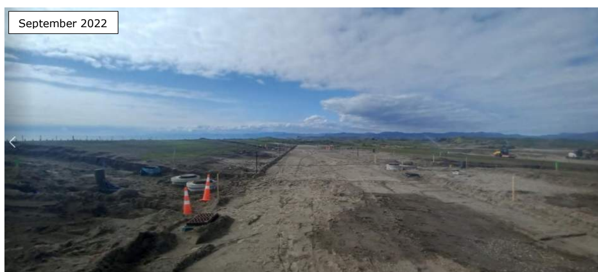
Figure 9: Subgrade and subbase for the RoW and road for Stage 5B
