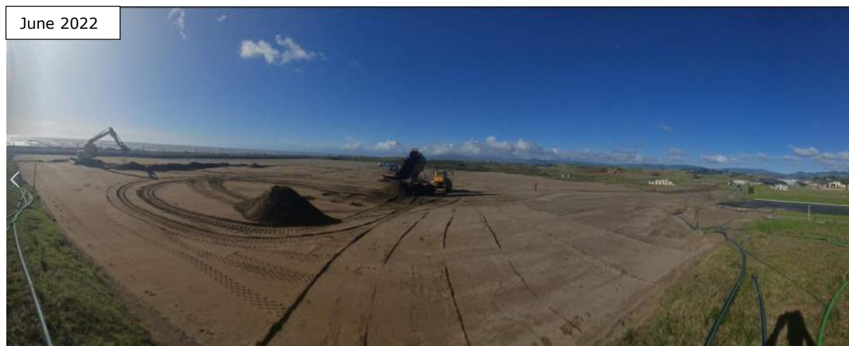
Figure 7: 1 st Compaction Inspection for Stage 5B
