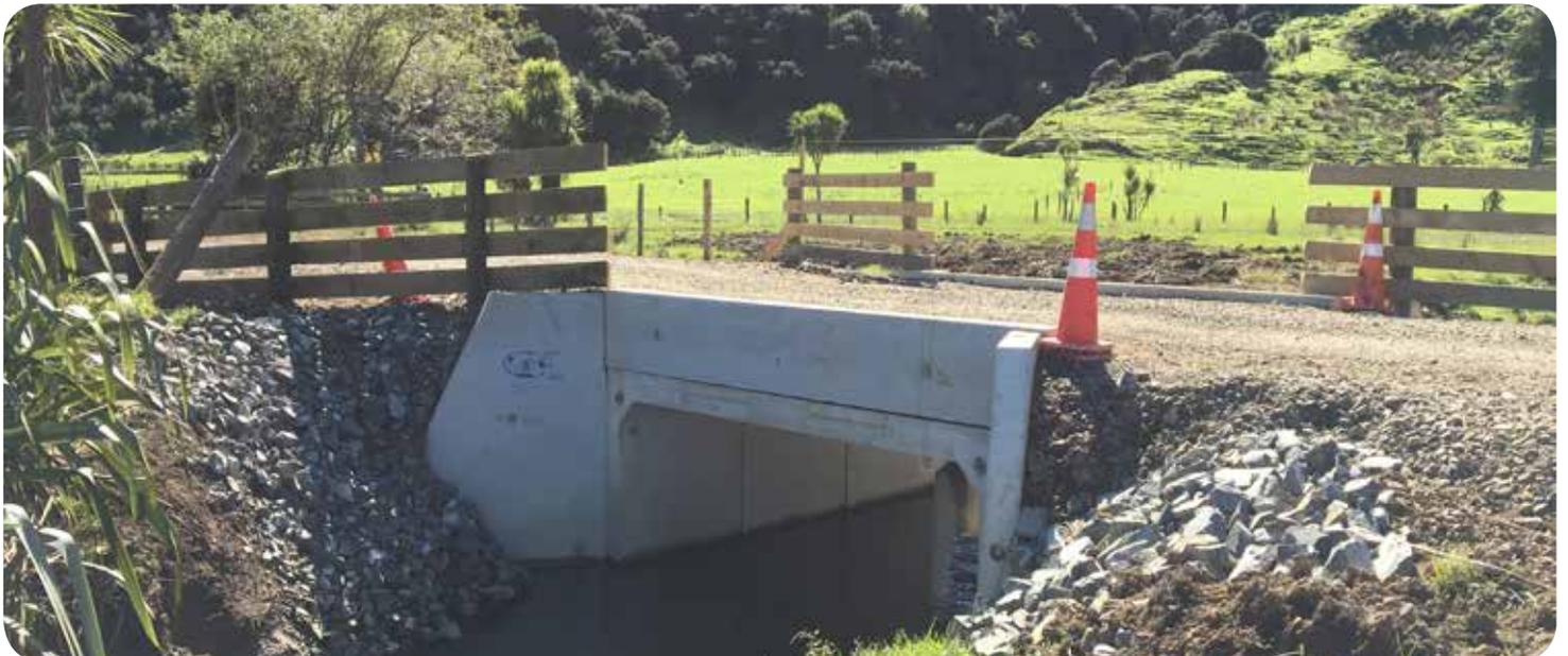
A full bridge replacement was included in the recent Long Term Plan and, earlier this year, the old bridge was replaced with a simpler concrete box culvert.
