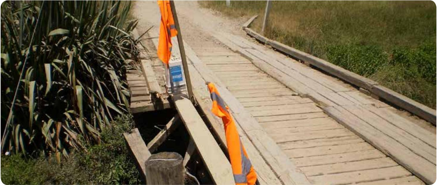
The old bridge was built in 1947 of wooden piles, steel beams and a timber deck. It had a fairly tough life. Being just over 12m long and single lane it was in constant need of repair from damage sustained by larger vehicles entering and exiting.
