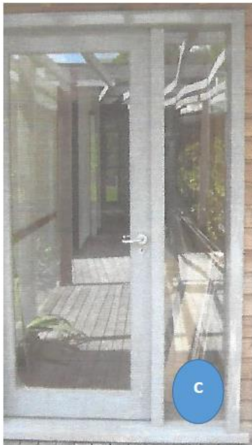
East-side exterior Door C Door 1m w and 2m high Faces Covered Disability Ramp Entrance
