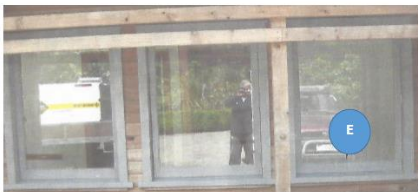
West-side face F Window, fixed leadlight Approx .800 wide x .400 high Serves to let some afternoon light into Pantry area
