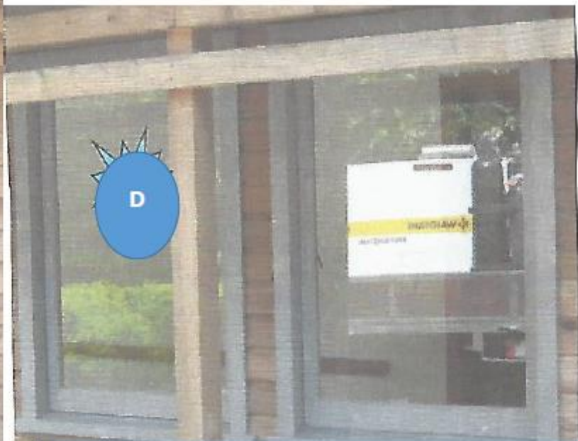
South-side D: A pair of push-out windows on the South/West corner above kitchen bench Each window approx .600 wide x 1m high
