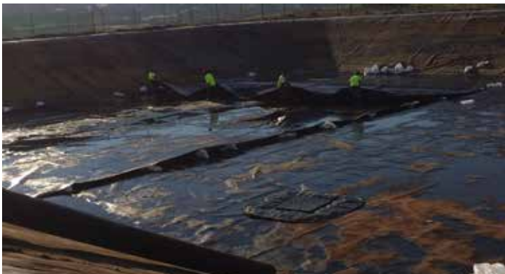
Step 2 – Take up the old liner in pieces. It is heavy work!
