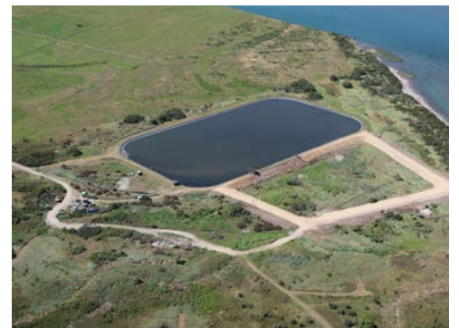
Aerial photo of the new and improved overflow pond.
