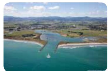
These twin seawalls will provide a year-round navigable harbour entrance to be used by a wide range of craft with a strong focus on servicing the growing mussel industry right on our doorstep. This will allow fresh produce straight to the planned processing factory here in Ōpōtiki.
